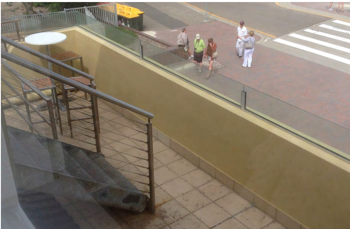
Figure 4.18: View showing the open space behind the parapet at the front. This area is at a lower level and was not originally linked to the sunbaking terrace. The highlight windows in the front wall of the hall open onto this terrace. The level of the parapet has been raised with glass panels, presumably for safety. The current stair is in a different location to that shown on the 2005 drawings but the location may have been changed during construction. Source: Jean Rice Architect
