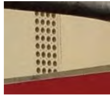
Original 'cast cement ventilating panel' or grille to rear stair which allowed fresh air into the staircase. Source: Jean Rice Architect
